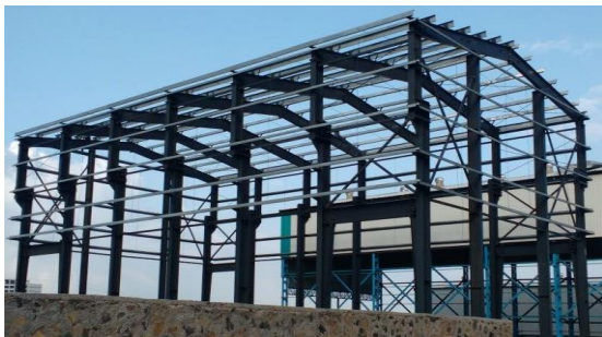
Project In process photo
