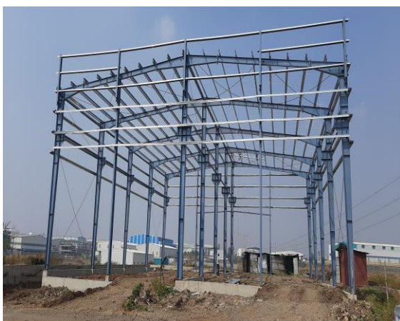
Project In process photo
