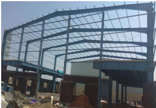
Project In process photo
